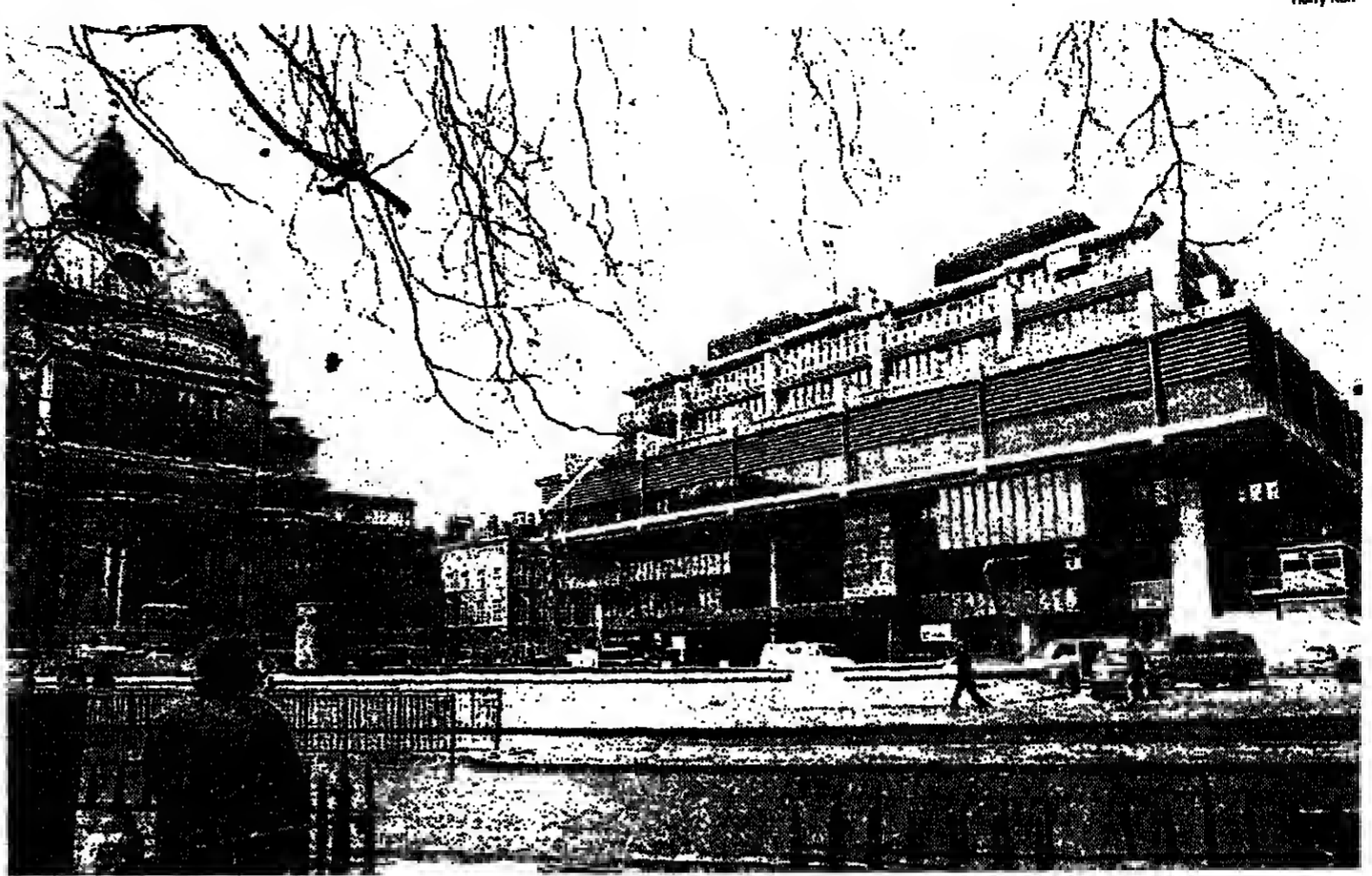
The new Queen Elizabeth II conference centre: Built by the Government opposite Westminster Abbey and near Parliament Square
